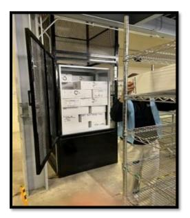
**Note:** Maximum capacity of dumbwaiter is 500 pounds; use caution as you are loading to prevent possible overloading. If the boxes seem overly heavy, split the delivery into two trips.
